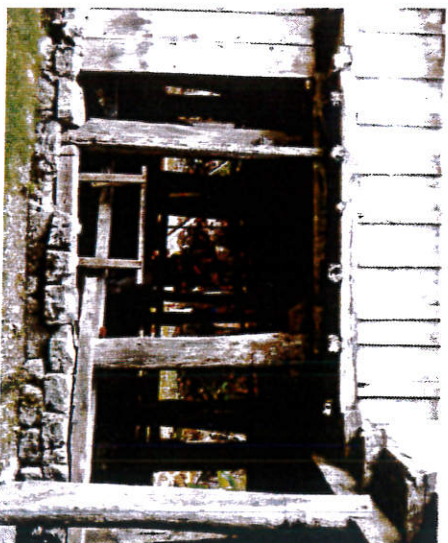
View of the 'silong' of the structure.
